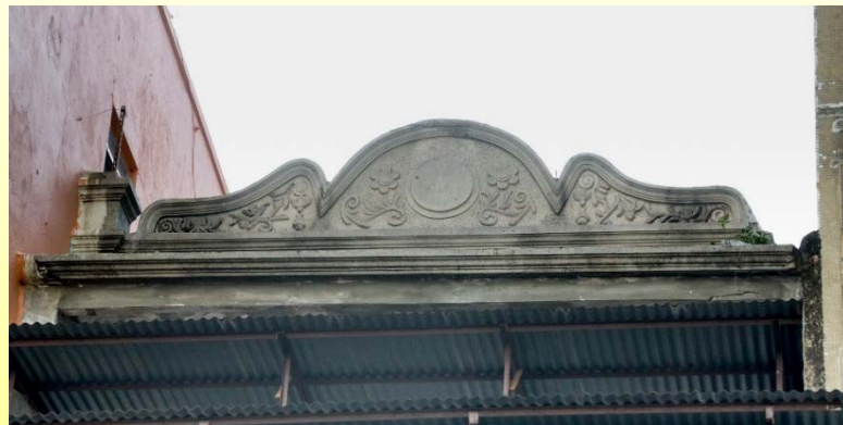
屋頂矮牆 Roof parapet
